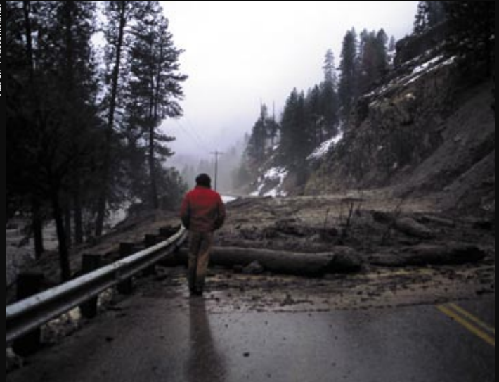
Erosion – mass wasting or debris flow.
