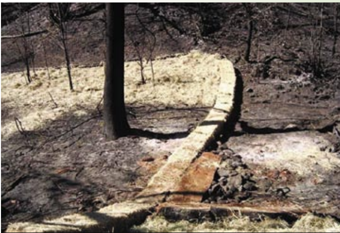
Straw bale check dam.
