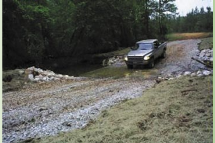
Armored stream crossing.
