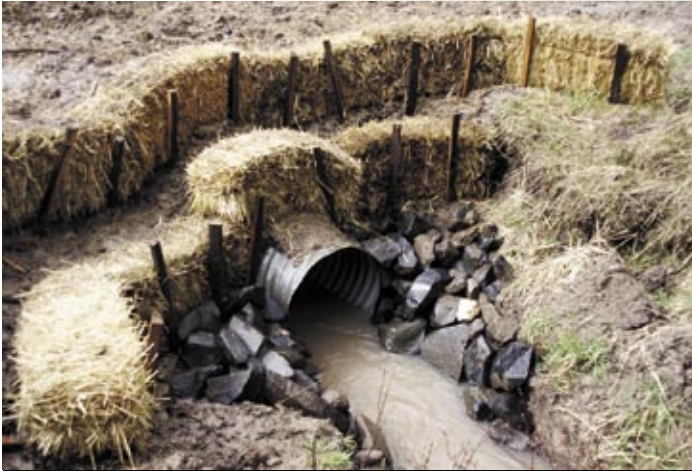
Properly installed and protected culvert.
