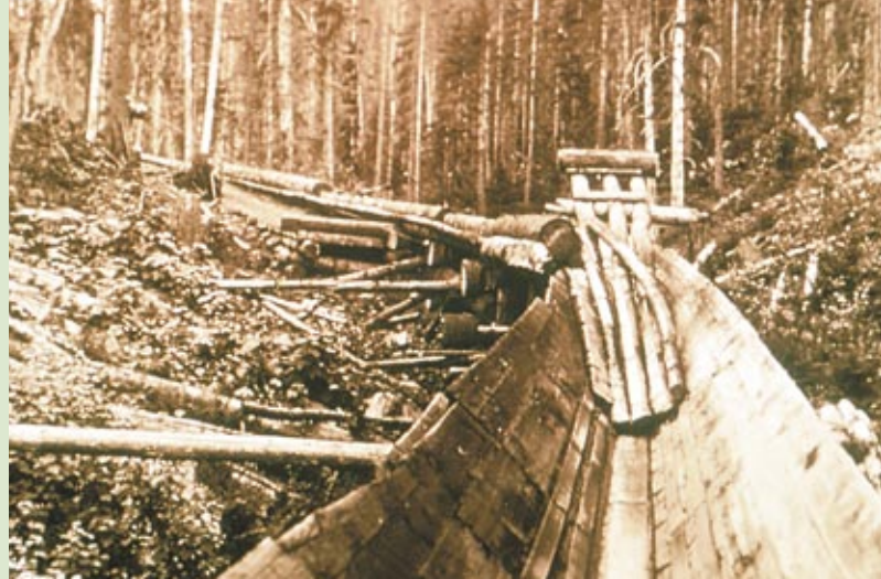
Logs being moved downhill in a flume.
