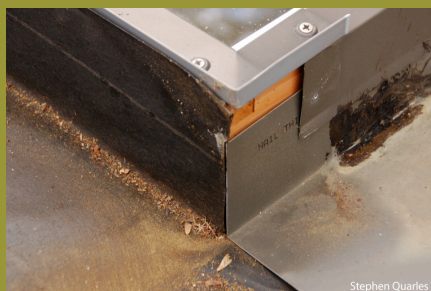
Photo 4. Metal flashing protects the framing members of a skylight from moisture, a direct ember ignition, or flames from ember-ignited vegetation debris.
