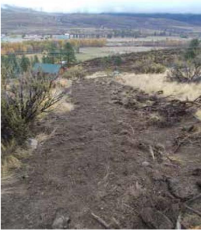
A fireline with removed material pulled back onto the disturbed soil.
