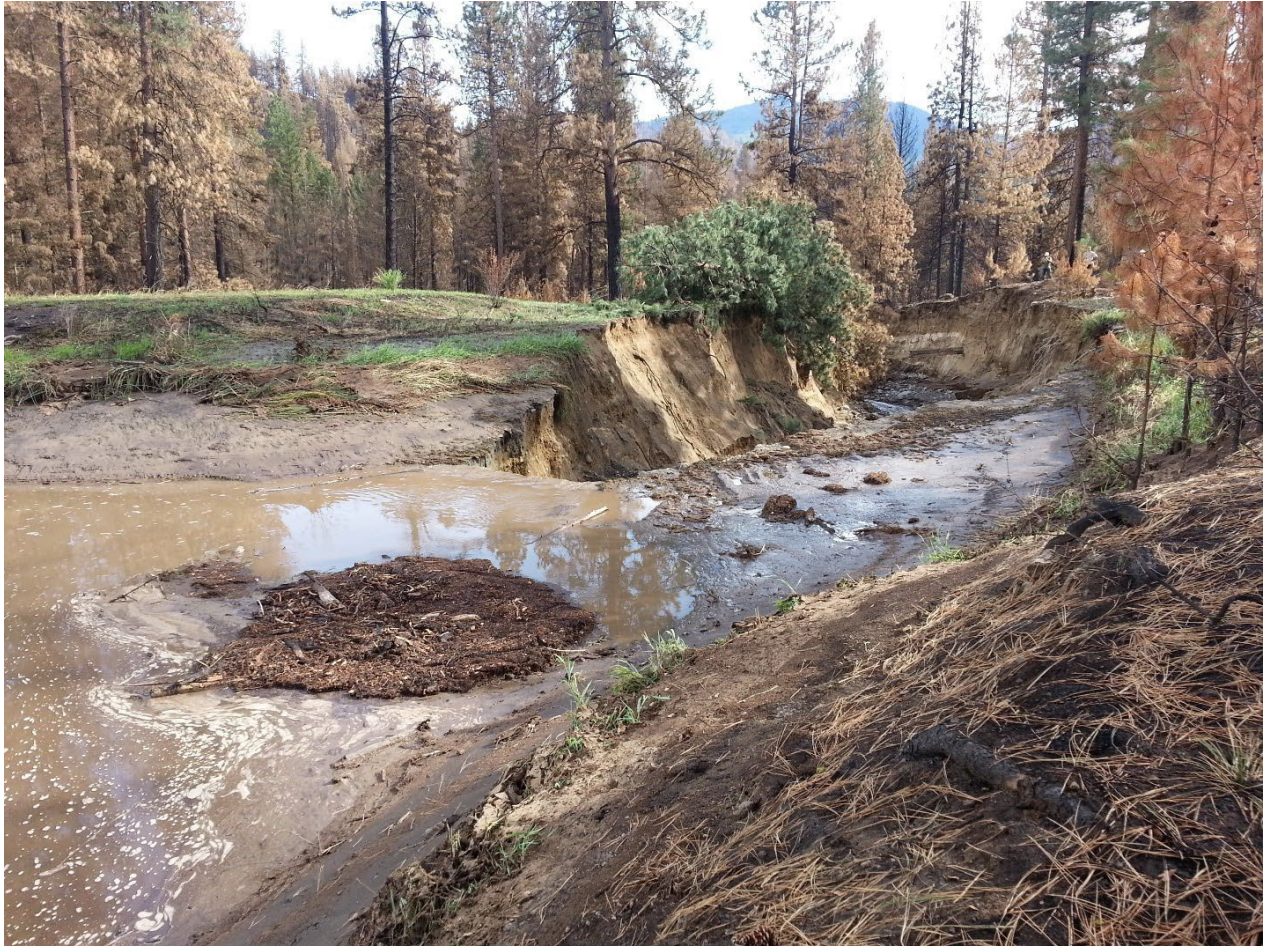
Figure 3.d.2. Post-fire flooding damage. (Source: Okanogan CD, 2014)
