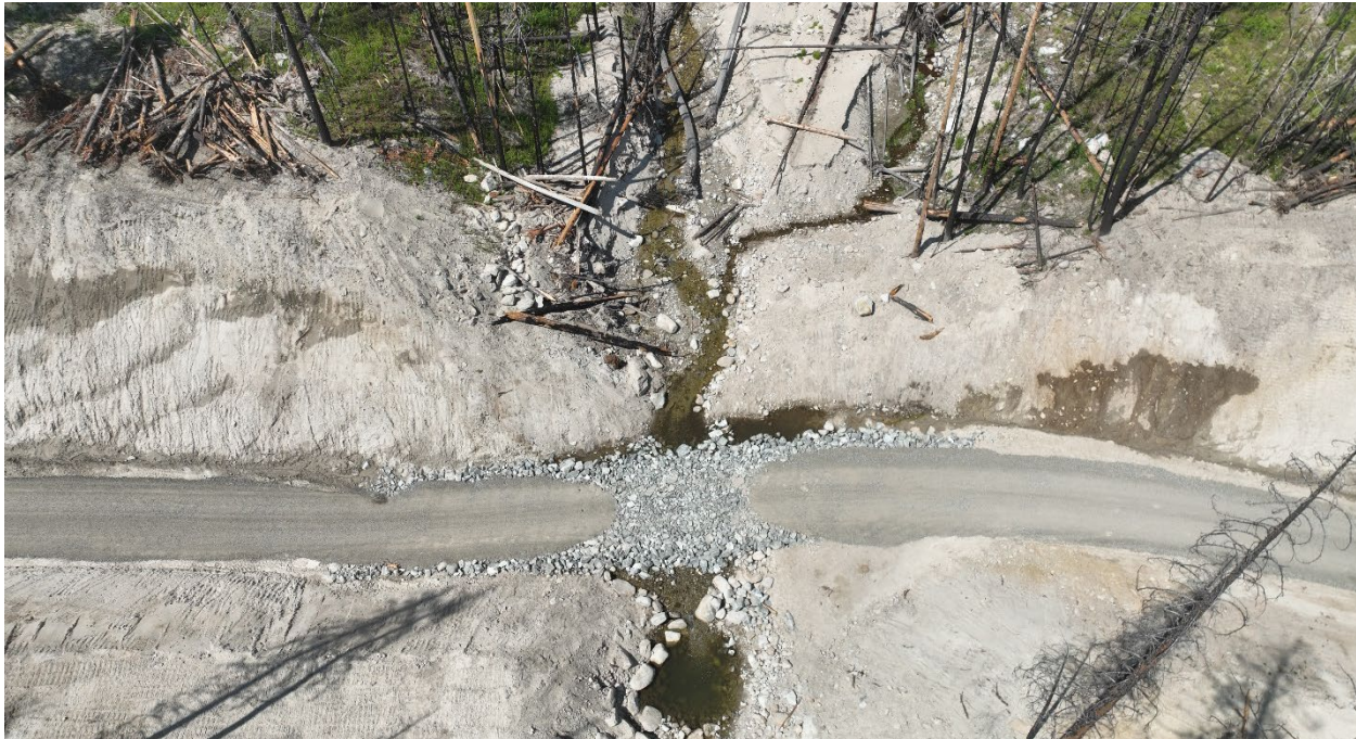
Figure 1.b.10. Debris flows, floods and other post-fire hazards can require significant effort to mitigate and possibly obstruct future firefighting efforts. This crossing was constructed by the Tonasket Ranger District in the aftermath of repeated blowouts of Lightning Creek in the Okanogan Highlands after the 2021 Walker Creek Fire. (Source: Mike Baden, WSCC, 2024)
