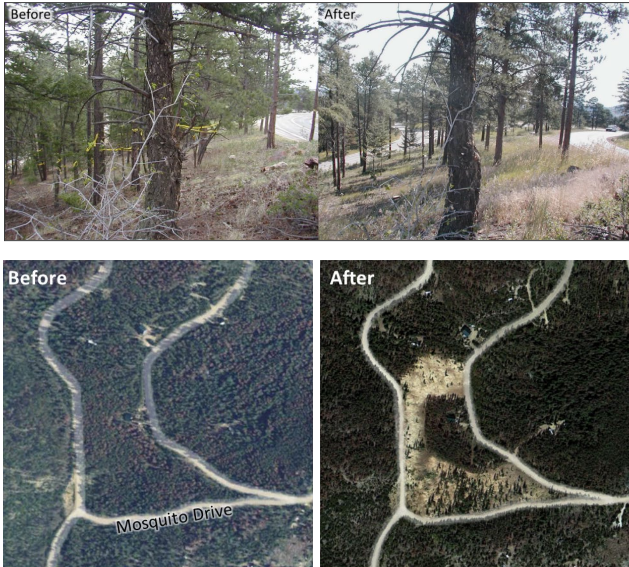
Figure 6.a.2. Effective roadside fuel treatments remove enough trees to result in widely-spaced crowns, remove ladder fuels (seedlings, saplings, shrubs, and low limbs), and reduce surface fuels. More dramatic tree removal along roadways can create even safer roadside conditions where appropriate.
