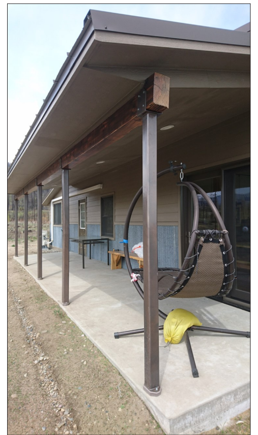
This home exemplifies fire resistant construction with its metal roof, metal and fiber cement siding, concrete perimeter, and metal posts.
